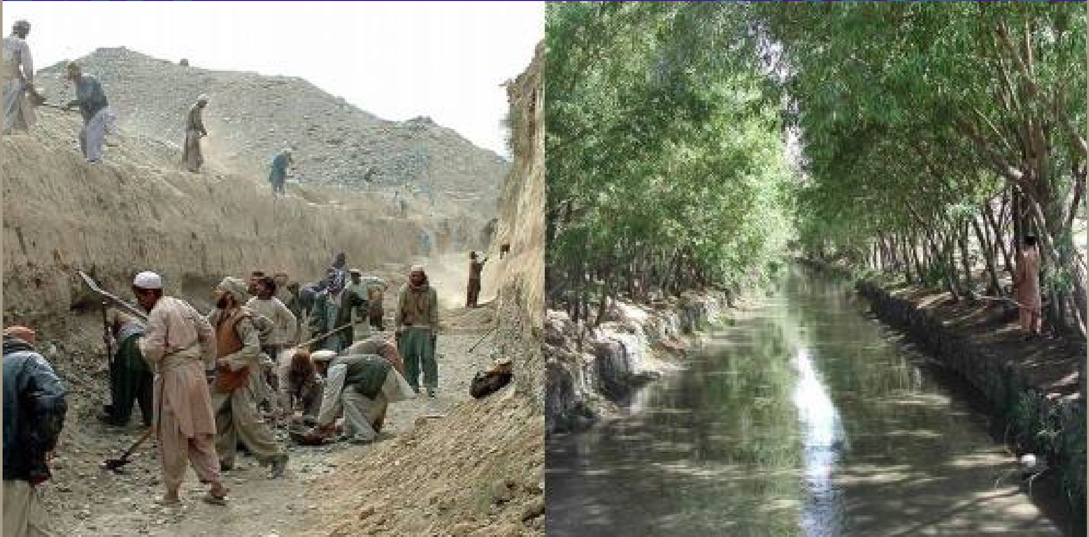
The irrigation canal during construction and after completion ( Peshawar-pms.com )
